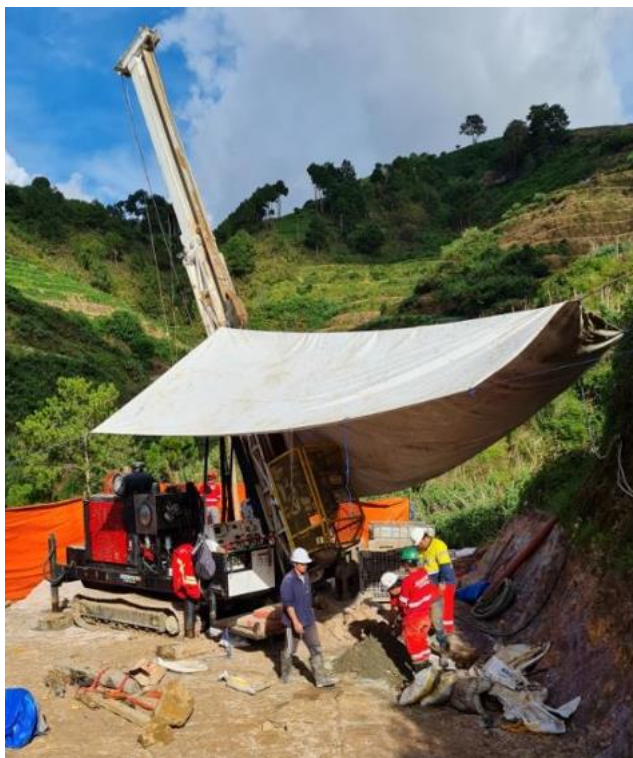
Figure 9_3 IDM Drilling 2022 - Major Drilling rig CDH-061 (Source: IDM, 2022)
